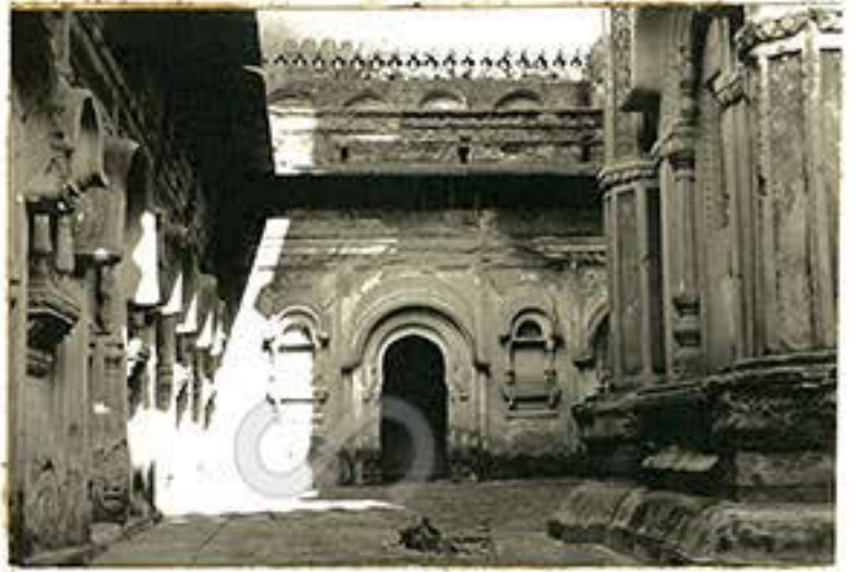
Ground floor- courtyard
